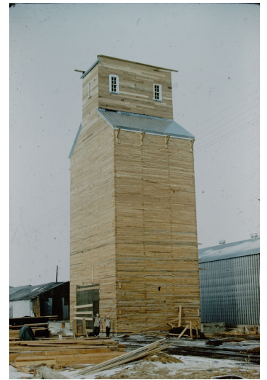
Wood Cribbed Elevator built in Union, IA
