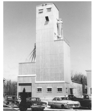
T&S's First Steel Feed Mill built for Goodman Milling in State Center, IA
