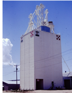
T&S's First Concrete Feed Mill - 1969
