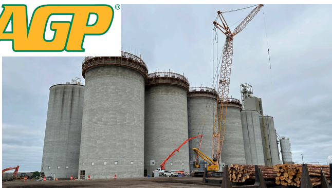
AGP // Storage Expansion Port of Grays Harbor, Aberdeen, Washington
