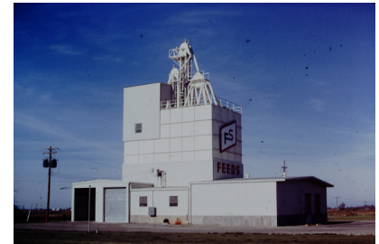
T&S continued constructing steel mills after beginning slipform, such as this mill in Alpha, IL, built in 1970
