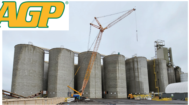
AGP // Grain Storage Expansion Port of Grays Harbor, Aberdeen, Washington
