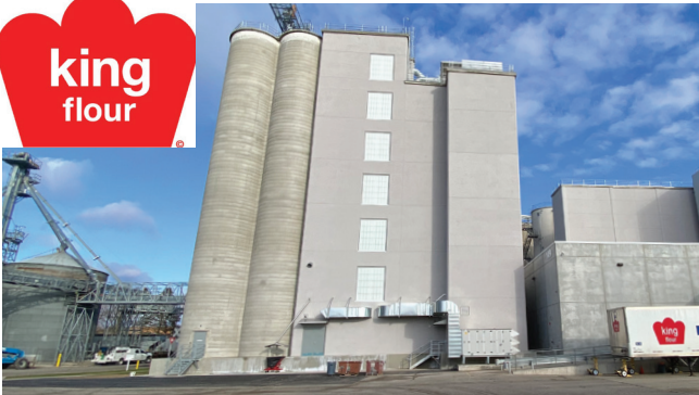
King Milling // Flour Mill Expansion Lowell, Michigan
